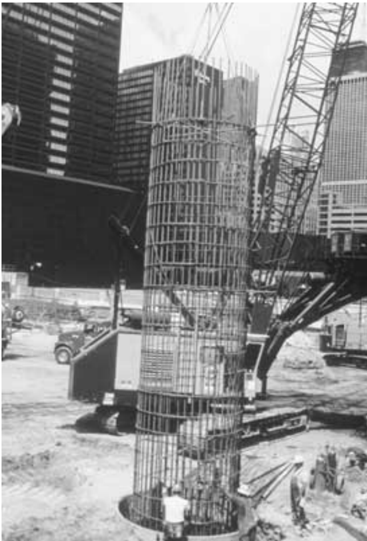
Installation of reinforcing steel for 9'-6" \Phi tower caisson.
