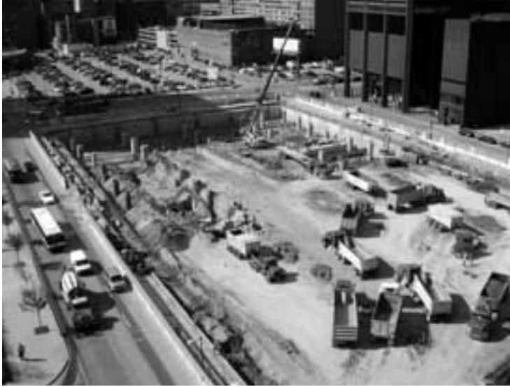
Mass excavation to parking level 1 at -15'. Slurry walls in place.
