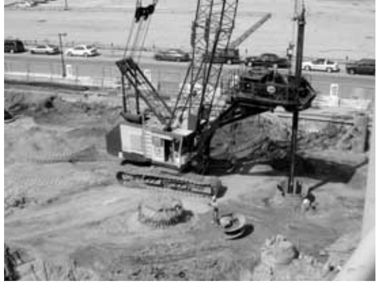
Caisson Installation. Completed 9'-6" \Phi tower caisson in foreground.
