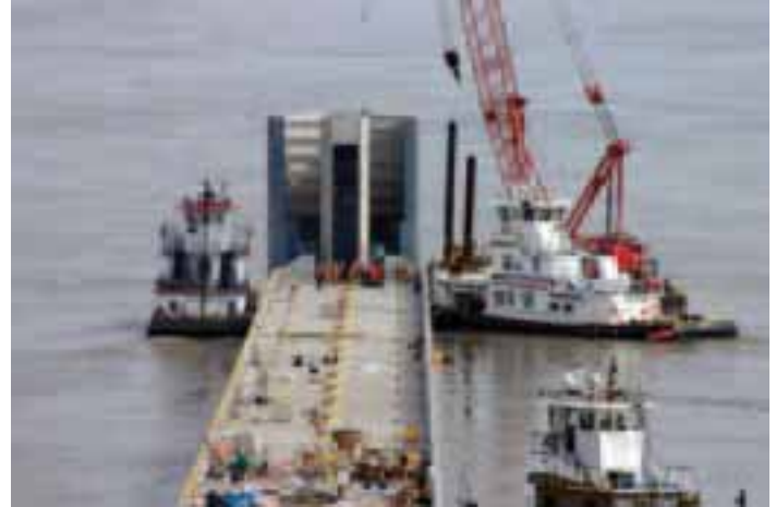
Figure 8 – Final Installation of the Floating Approach Wall
