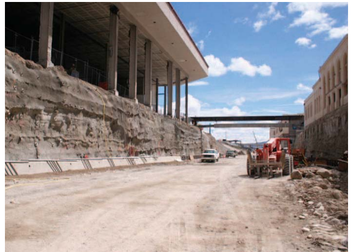
Figure 8. Micropile Underpinning of Bowling Stadium (left side)
