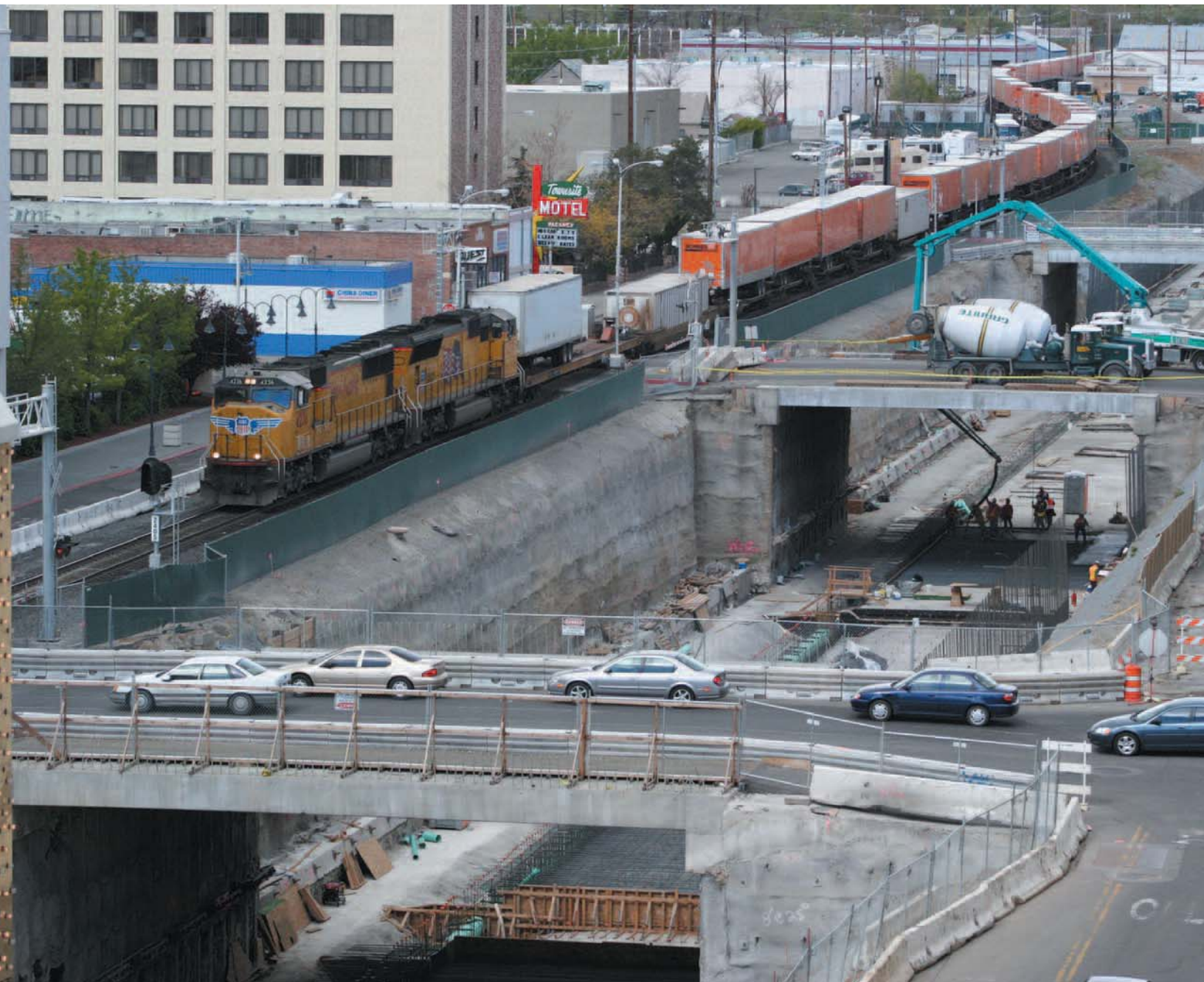
View of ReTRAC Trench spanned by temporary bridges, showing soil nail and shotcrete retaining wall subjected to Cooper E-80 train loading from shoofly
