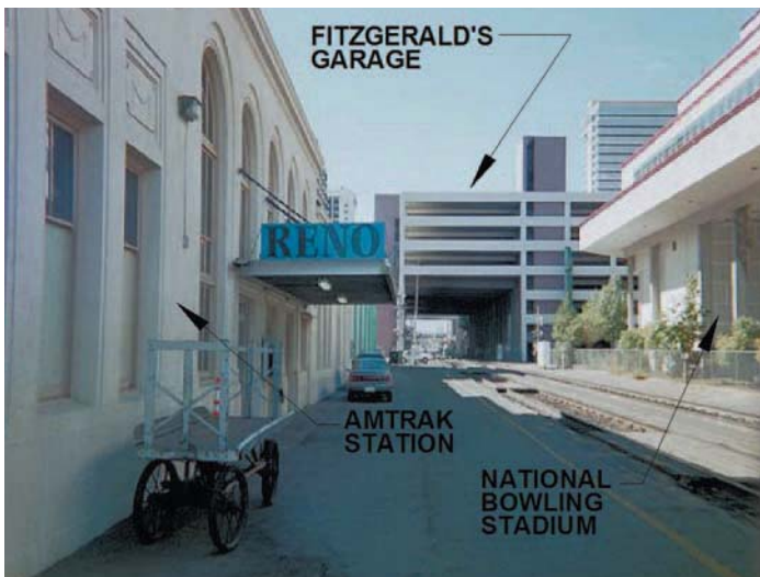
Figure 2. Preconstruction Condition Looking West
