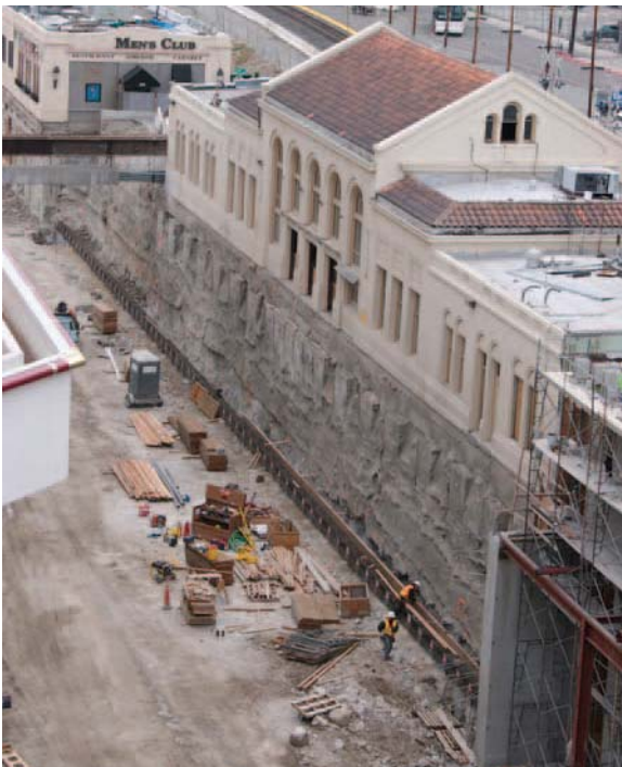
Figure 7. Micropile Underpinning of Historic Amtrak Structure
