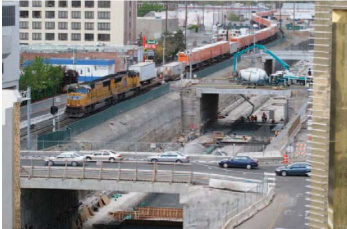
Figure 9. Soil nail shoring to protect railroad shoofly
