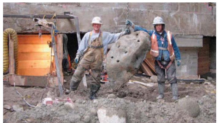
Figure 4. Boulder removed from pit
