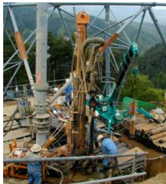
Photo-6.5 Appearance of construction
