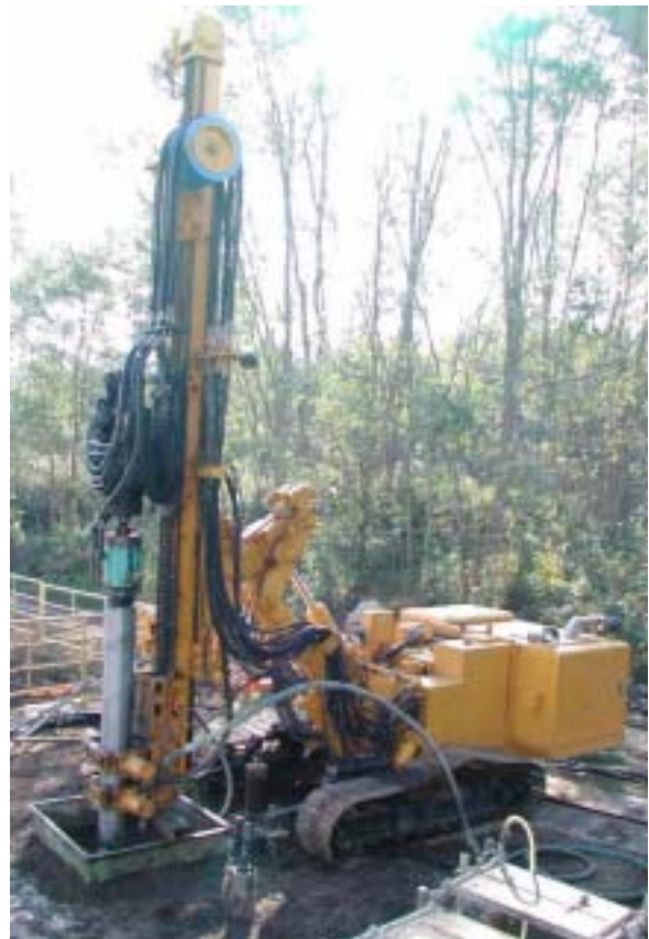
Pohto-7.1 Appearance of NEW-HMP construction
