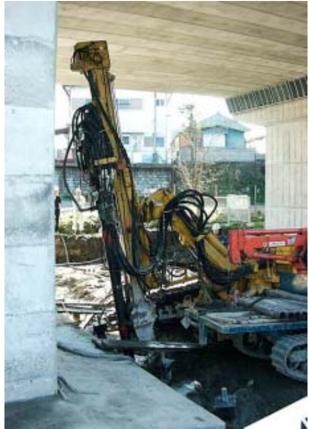
Photograph-6.1 Appearance of construction
