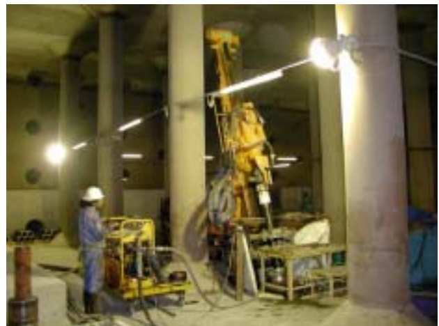
Photo-6.2 Appearance of construction
