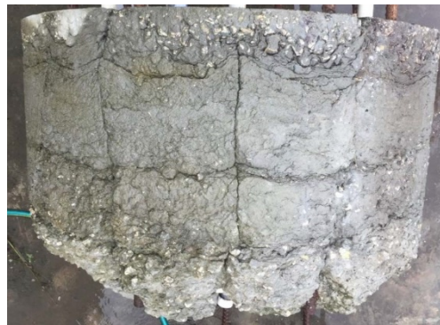
Figure 3: Mattressing in a drilled shaft
