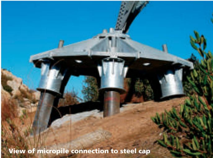
View of micropile connection to steel cap
