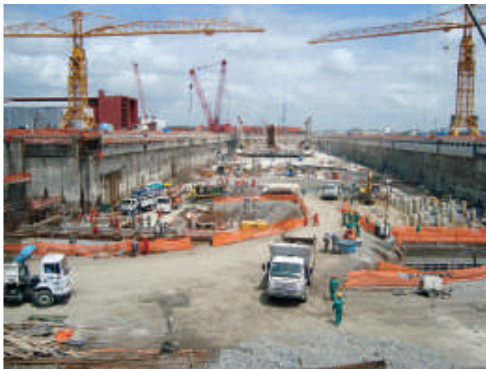
Construction underway for the dock floor
