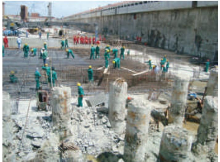
Piles rising from the dock floor
