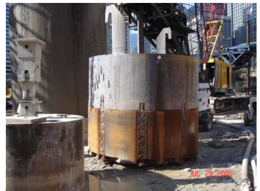
Cluster Drill at work on jobsite.
