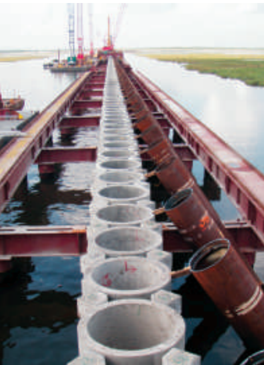
Completed floodwall foundation pile
